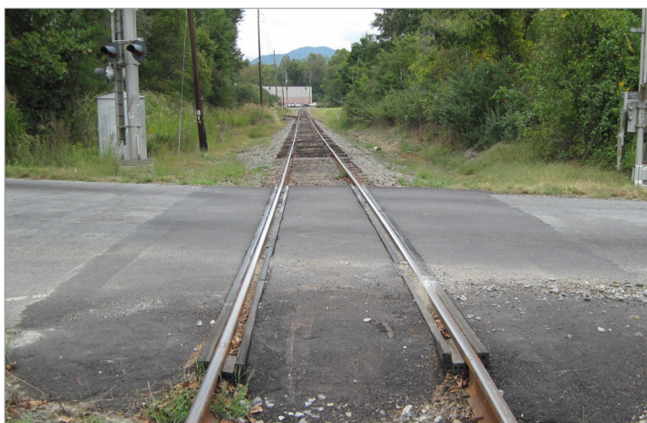
Cane Creek Road crossing after improvements
