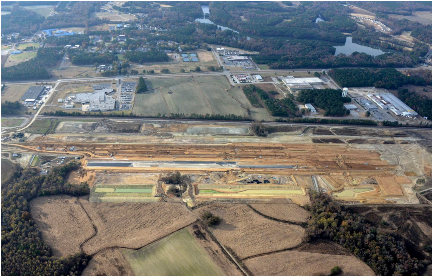
Aerial view of terminal site looking west
