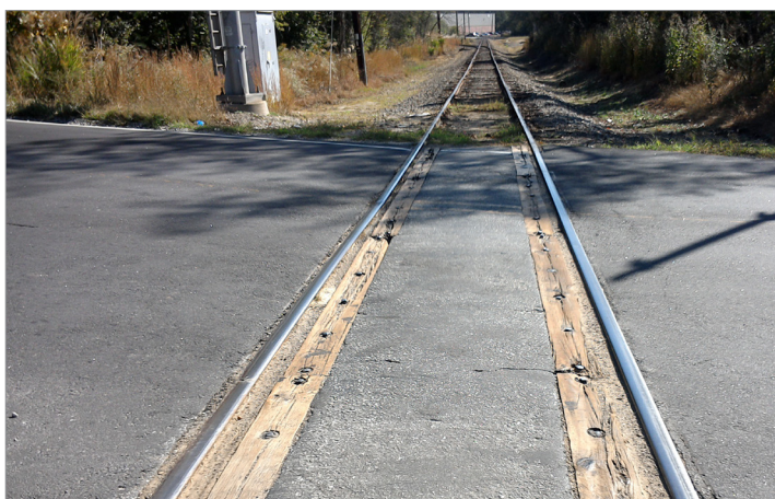
Cane Creek Road crossing before improvements
