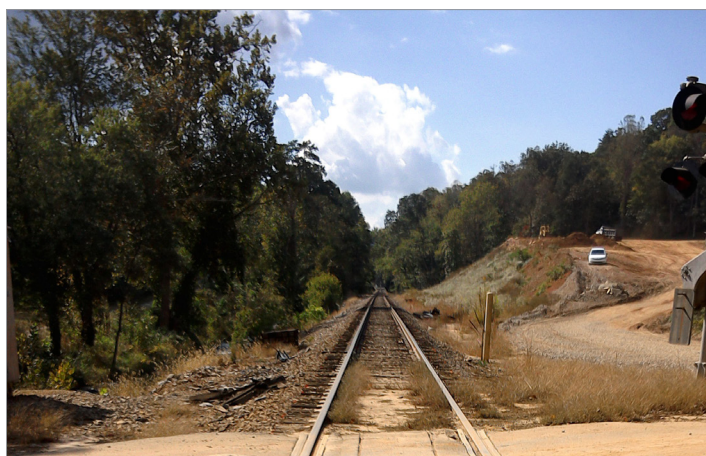
Hominy Baptist Church Road crossing before improvements
