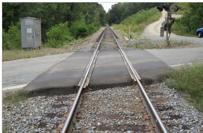
Hominy Baptist Church Road after improvements
