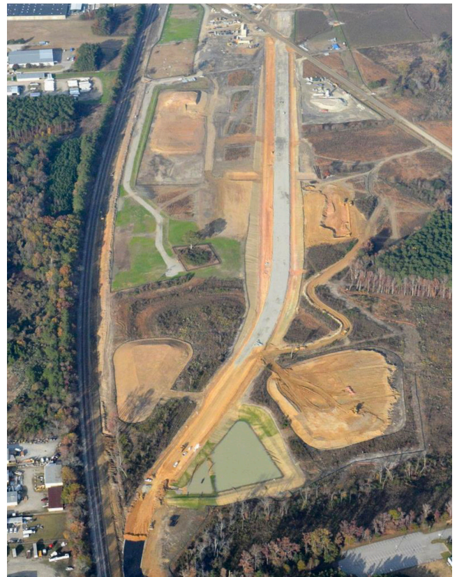
Aerial view of south lead tracks roadbed grading
