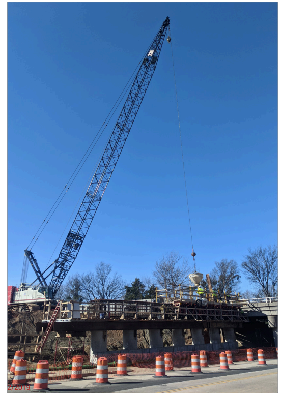
Pouring 4th Street bridge cap
